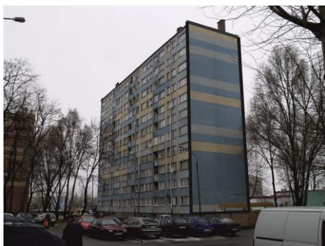
Fig. 1. Typical high-rise prefabricated apartment building
